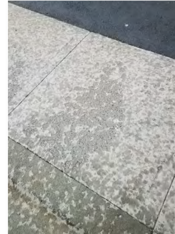
Concrete Spalling
