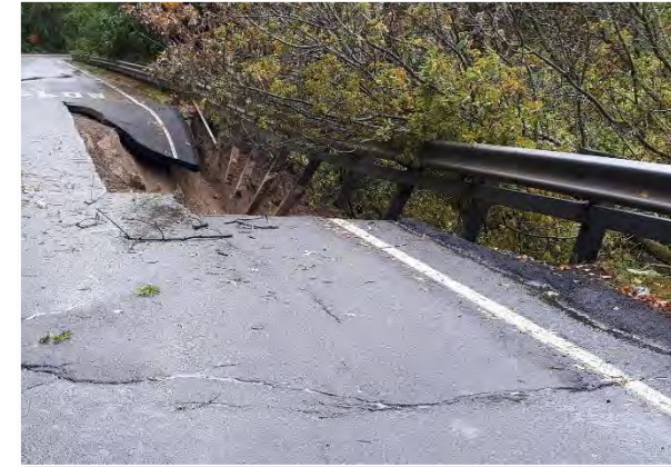
Hwy 8 Dundas Escarpment Failure
