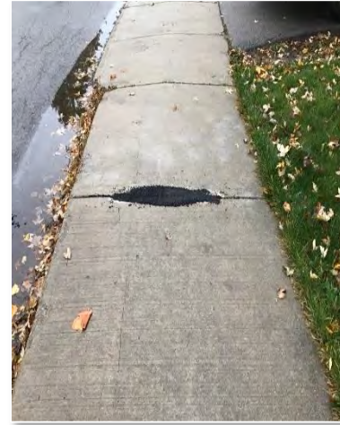
Asphalt Repair
