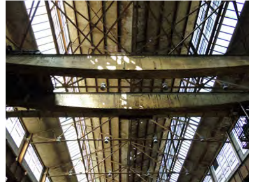
Production shed with butterfly roof, complex fenestration system and traveling crane, 2016 (ERA Architects)
