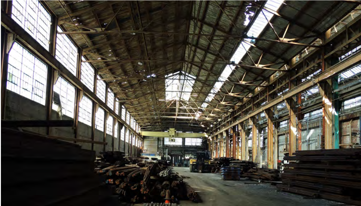
Above: Westernmost production shed, looking north. Note rows of flat skylights along pitched roof, extensive glazing along exterior wall, and overhead travelling crane at the shed's north end, 2016 (ERA Architects).
