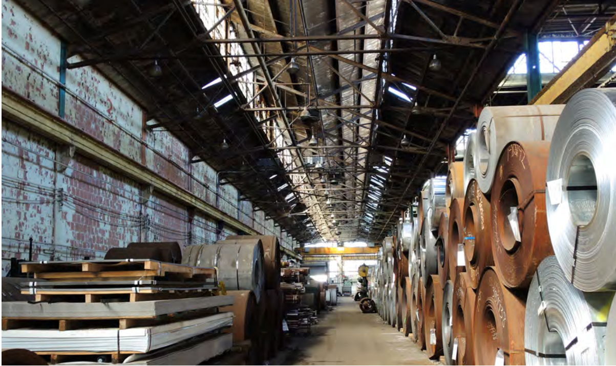
Above: Third production shed, with butterfly monitor roof, looking north. Note hollow tile structure of west wall. Below: Easternmost production shed, added between c.1924 and 1940, looking north. Note Aiken roof form with alternating high and low bays, 2016 (ERA Architects)
