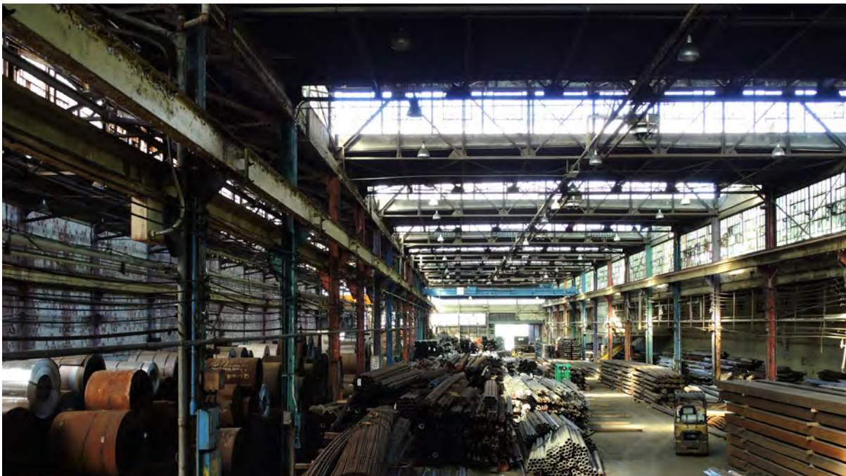
Above: Third production shed, with butterfly monitor roof, looking north. Note hollow tile structure of west wall. Below: Easternmost production shed, added between c.1924 and 1940, looking north. Note Aiken roof form with alternating high and low bays, 2016 (ERA Architects)
