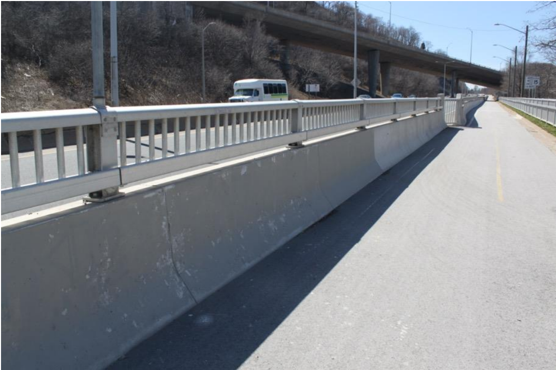
Figure 2: Example of Concrete Barrier Wall
