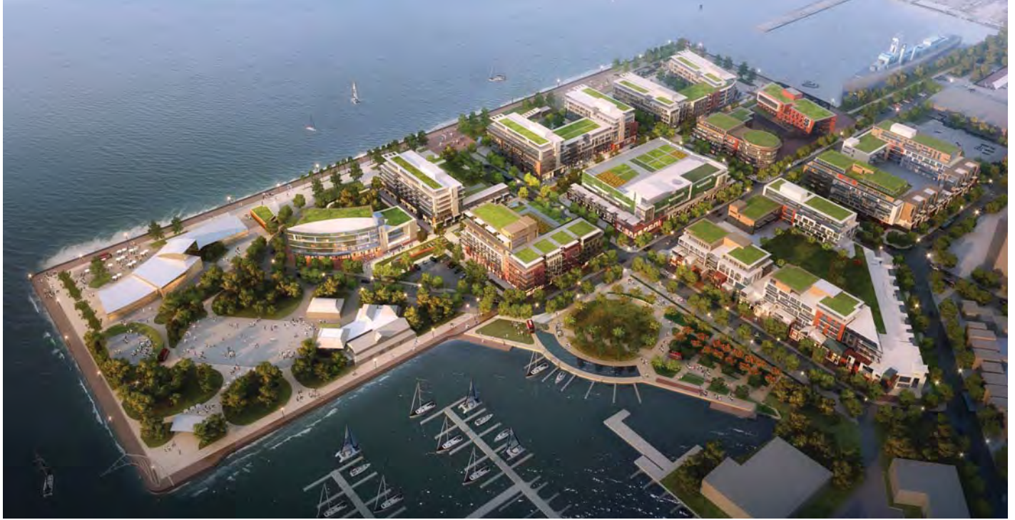
VIEW LOOKING NORTH - EAST
