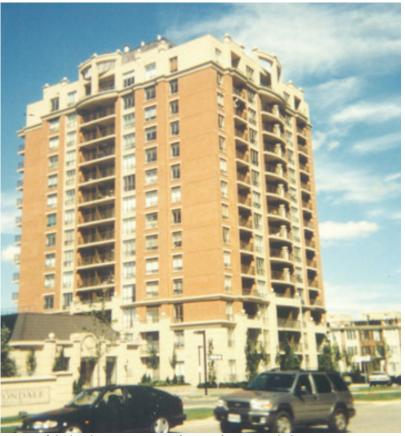
Roof design incorporates rooftop equipment and elevator penthouse to provide an attractive skyline
