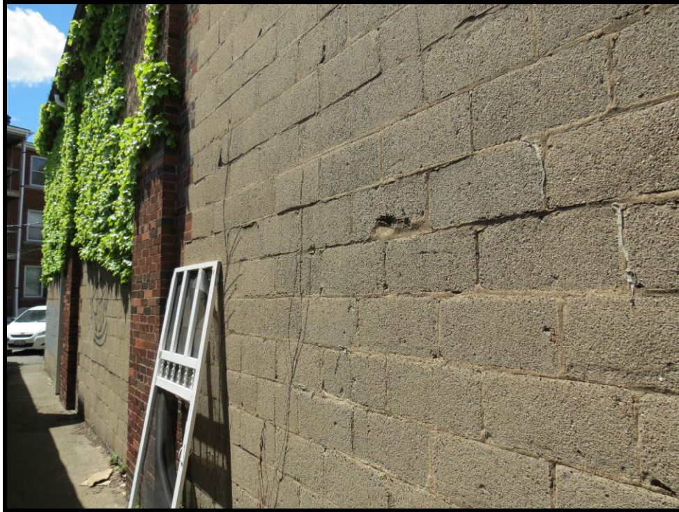
Image 6: South Elevation of 1014 King Street West, Hamilton – Westdale Theatre (Photo taken on May 29, 2017; Facing Northwest)
