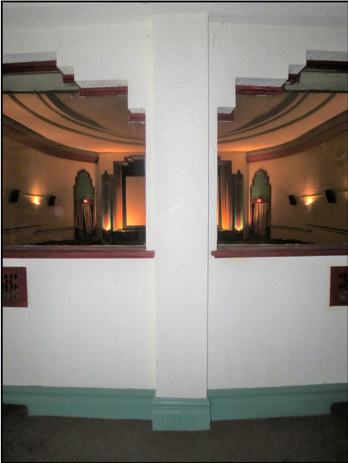
Image 33: Detail of column and window opening from the Foyer of 1014 King Street West, Hamilton – Westdale Theatre (Photo taken on May 29, 2017; Facing West)
