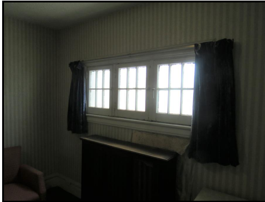
Image 25: Six pane wood casement windows in the Retiring Room portion of Ladies' Room of 1014 King Street West, Hamilton – Westdale Theatre (Photo taken on May 29, 2017; Facing Southeast)
