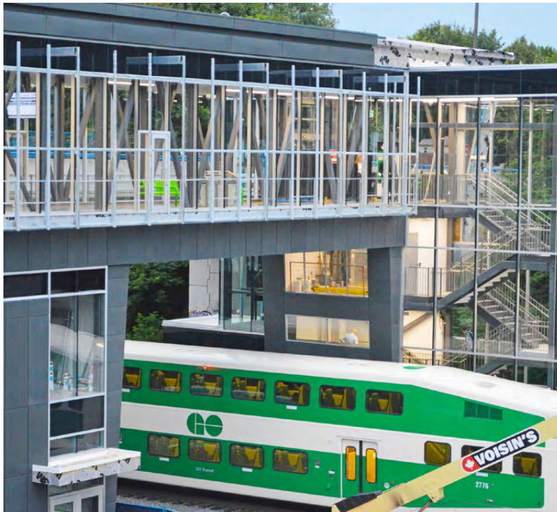
The new West Harbour GO Station (1 km from Pier 8)
