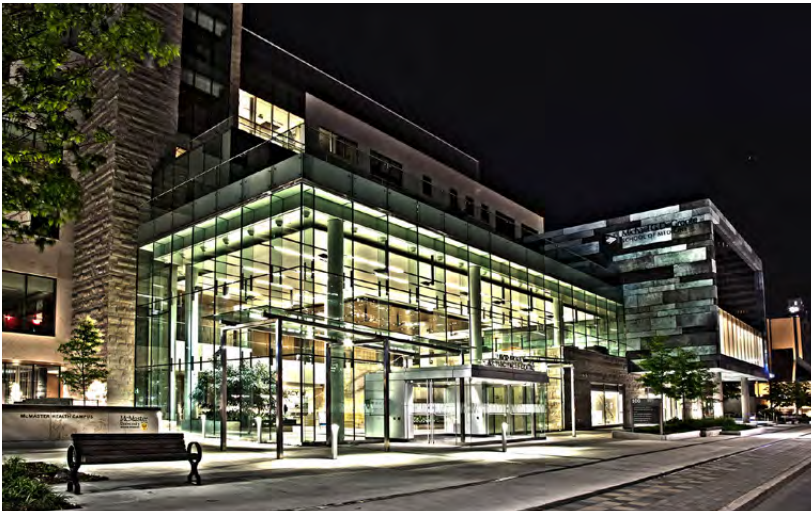
Braley Health Sciences Building is the new downtown campus for McMaster University's School of Medicine
