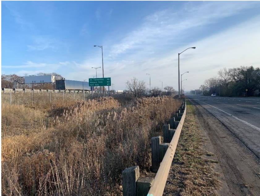
Plate 16: Looking south along Eastport Drive, view of the ditch to the left of the roadway (A.S.I., 2022).
