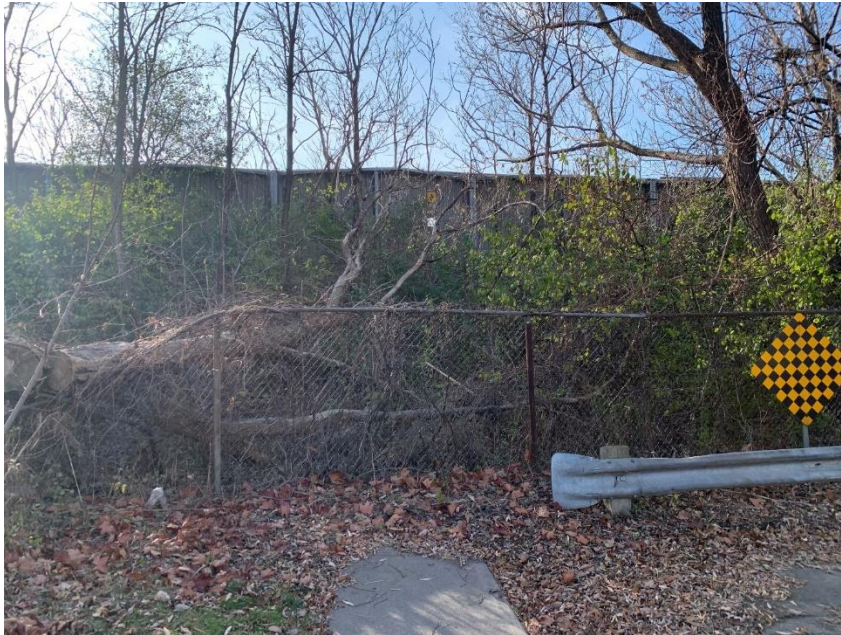
Plate 10: View of the Wark Outlet location, looking west at the western end of Wark Avenue at the barrier to the Queen Elizabeth Way (A.S.I., 2022).
