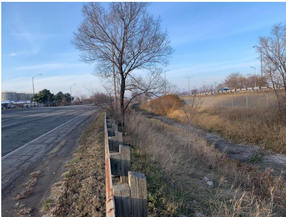
Image 6 Existing ditch rehabilitation between Eastport Drive and the Queen Elizabeth Way; Area is disturbed, no potential
