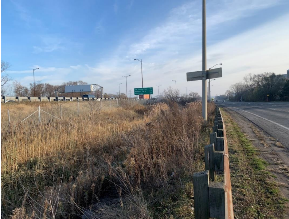
Image 7 Existing ditch rehabilitation between Eastport Drive and the Queen Elizabeth Way; Area is disturbed, no potential
