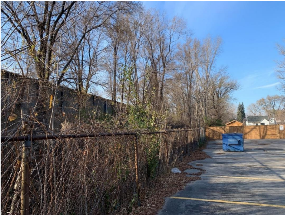
Image 10 east side of the Queen Elizabeth Way from Towers Drive to Van Wagners Drive; Area south of disturbed parking lot requires Stage 2 survey
